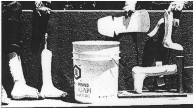
Photo of the steps in making Noé's plastic bucket braces.
