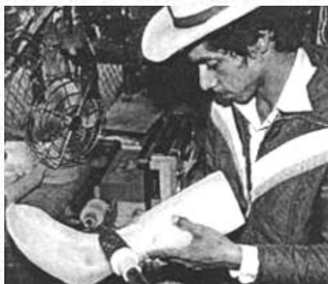
Marcelo is also a master craftsman, brace maker, and limb maker. Here, he makes a plastic leg brace.
