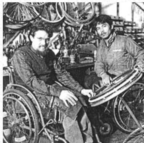
Ralf Hotchkiss examines the one arm drive wheelchair which Martín is building. The 2 hand-rims are on one side and can be powered together or independently with one hand.
