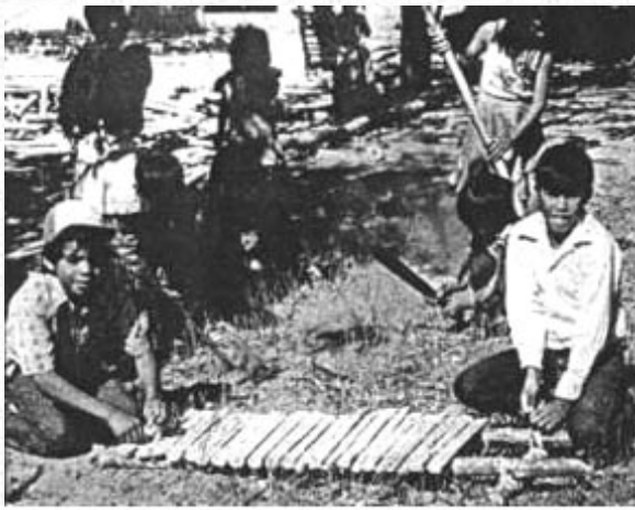
Out of poles they collected from the local forest, school children make a ramp as part of the equipment for the playground.
