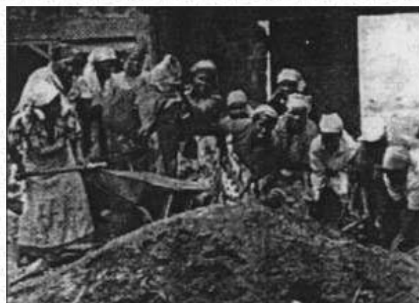
Mothers and grandmothers work together to build a cooperative bakery. Here they make mud bricks of earth mixed with straw.
