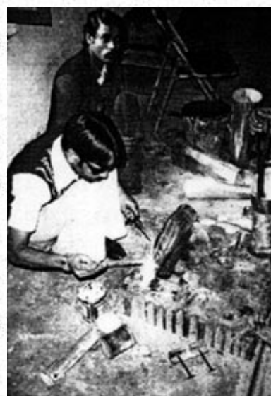
He welds the aluminum sheet into a tube.
